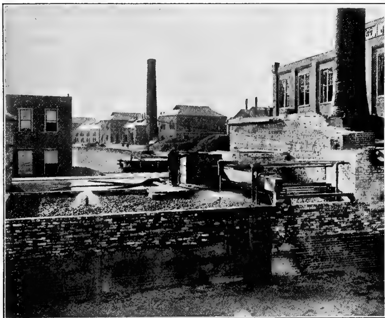
FIG. 117.—Sewage Experiment Station, Mass. Inst. Technology. Trickling filter in front, sand filter just behind filter, dosing tank just behind sand filter, and septic tank just behind dosing tank.
